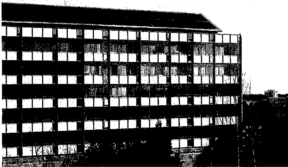
Roof module collectors on a renovated multifamily building in Gårdsten, Göteborg.
