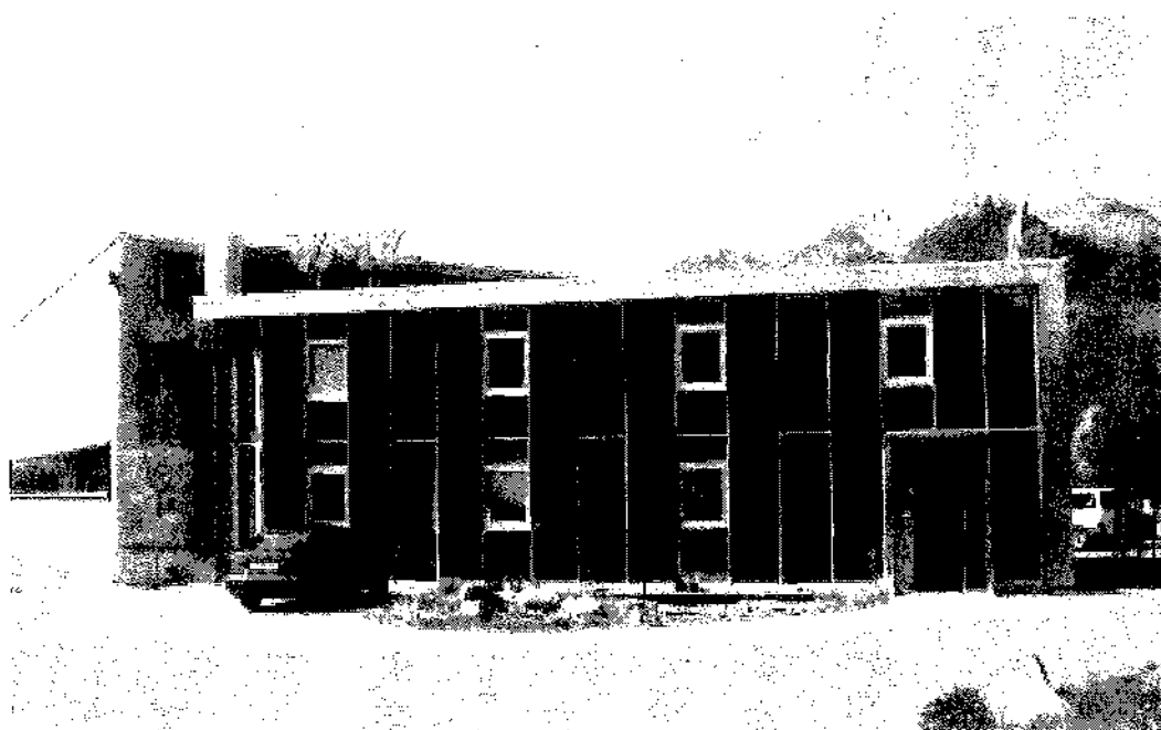
Fig. 3: Facade integrated collector at a commercial building (Source: DOMA)
