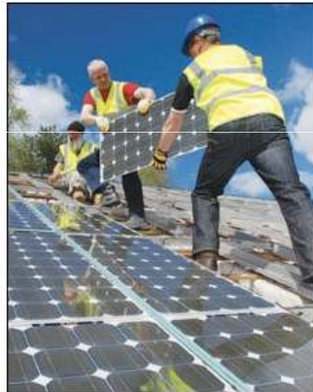
The report calls for every cavity wall and loft in the UK to be insulated
